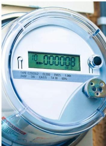
*For many years, electric meters have been the sole responsibility of electric utilities. Building owners are now installing their own electric meters to determine the power produced by on-site renewable energy sources, such as solar or wind. Green construction codes require a means for measuring, monitoring and reporting on energy use, production and reclamation in a building, which is accomplished by smart meters.*
